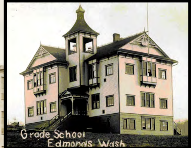
The 3-story Edmonds Grade School, now demolished, was built in 1891 to accommodate the town's mushrooming student population
